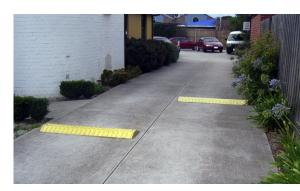
Recycled-plastic speed humps are flexible enough to allow them to conform to slight irregularities in the pavement surface, yet are strong enough to withstand reasonable loads. With a weight of 16 kg, Replas speed humps are light enough to be installed by one person without the use of lifting equipment.
