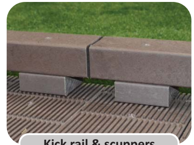
Kick rail & scuppers
